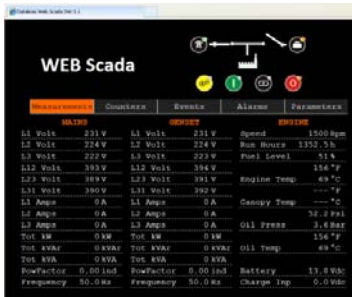
Monitoring and Control
